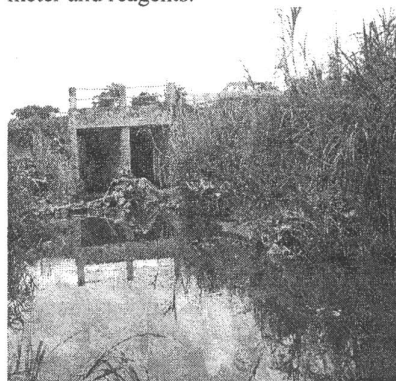
Figure .2b: River after effluent mixture
