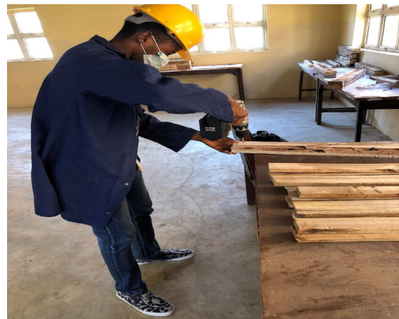
Fig. 6: Drilling holes for bolt-laminated beams
