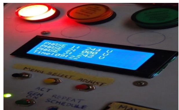
Figure 17. The front view of the constructed micro-controller-based automatic change-over.
