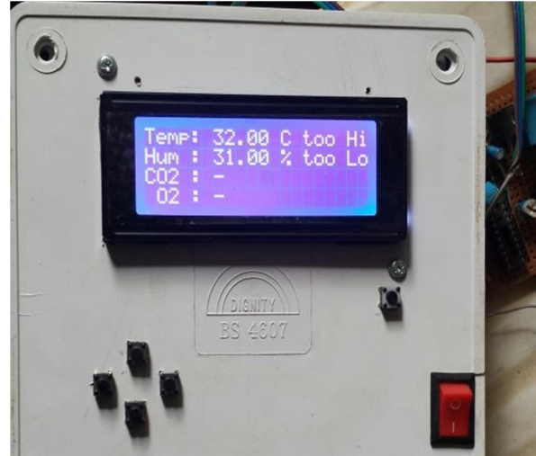
Fig. 6: The LCD when the DHT11 sensor was exposed to ambient temperature
